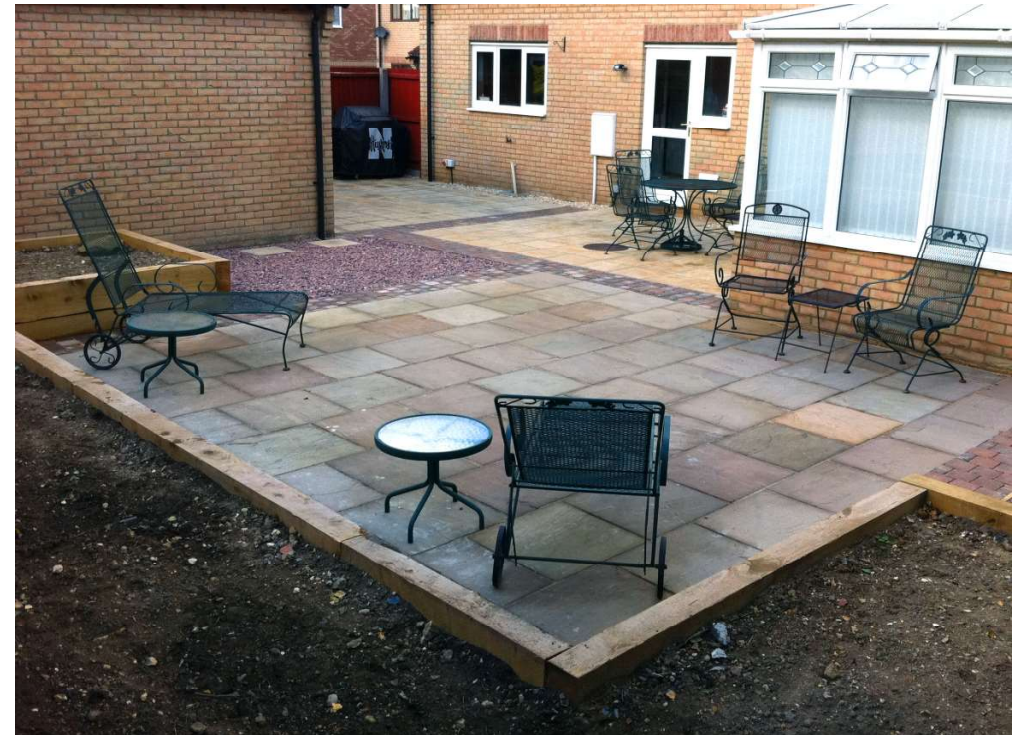
After - Completed New Terrace Garden.
