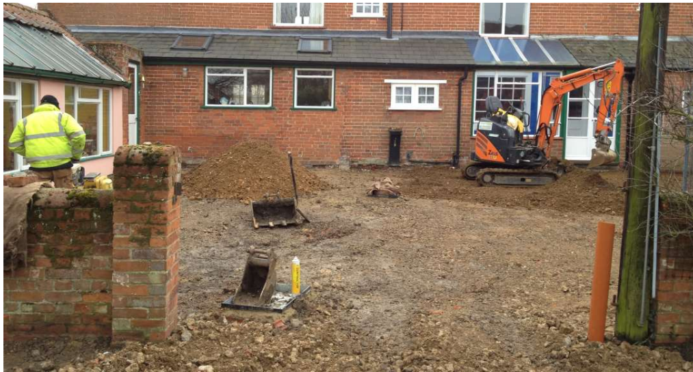
Garden During Construction.
