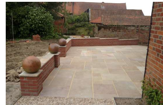
Garden After Completion.
