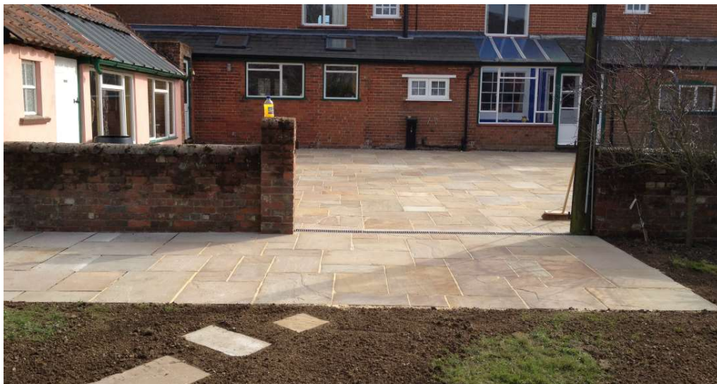
Garden After Completion.
