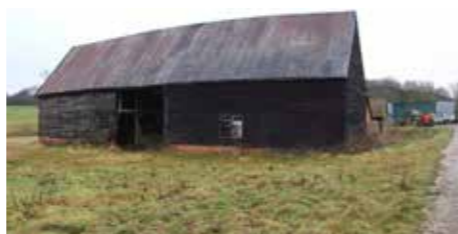
Existing Driveway & Medieval Barn.
