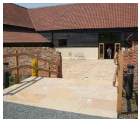
Inner Courtyard, After Completion.
