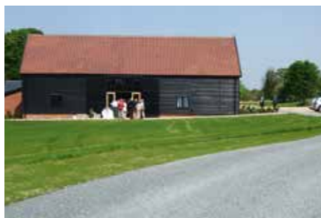
Driveway & Barn After Completion.
