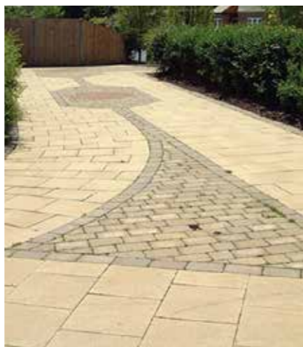
Crossing Point Paving Detail.
