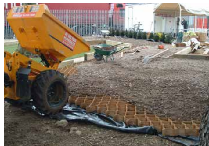
The Process of 'No Dig' Construction Around Existing Trees.
