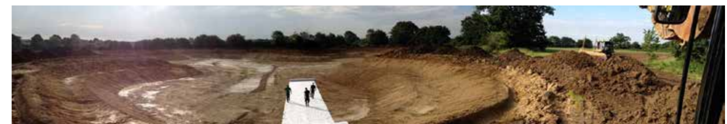
Lake Excavation and Liner.
